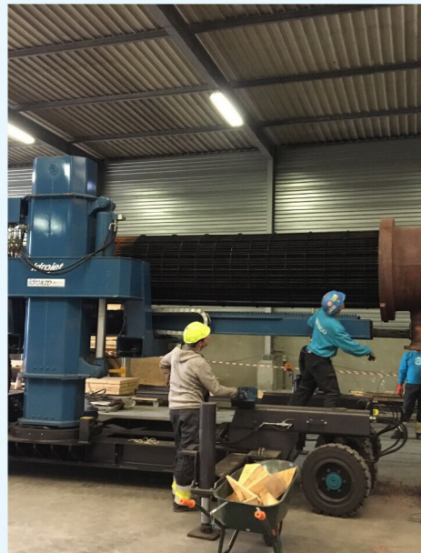
Step 4 Extract the tube bundle
