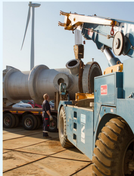
Step 1 You remove or swap out a complete heat exchanger
