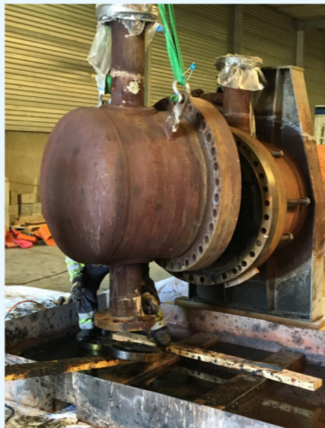
Step 3 Disassemble the heads and floating heads, among other components
